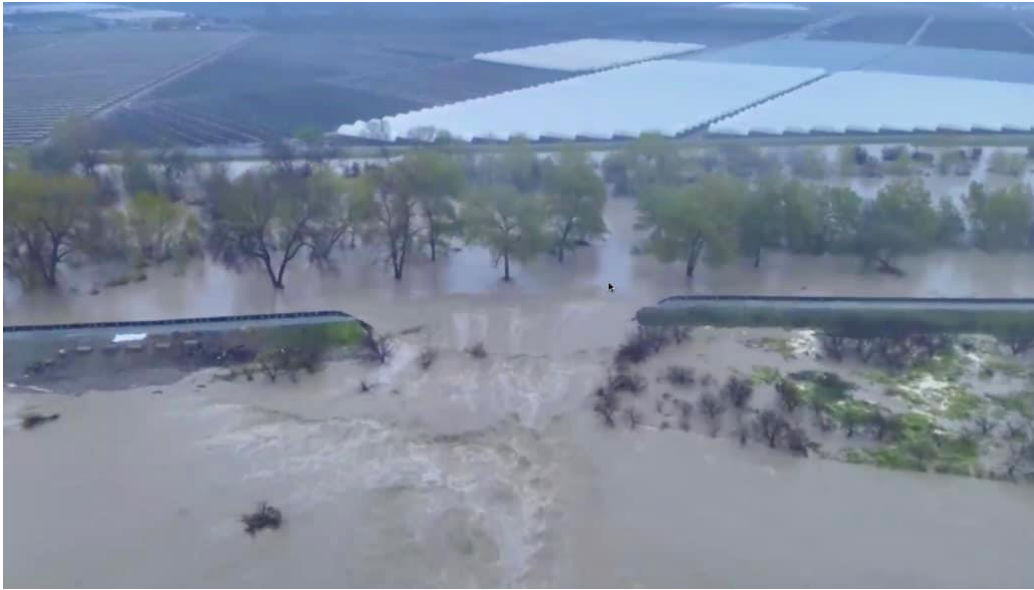
Figure 1: Levee Breach in Pajaro, CA caused catastrophic damage to homes on March 11, 2023
